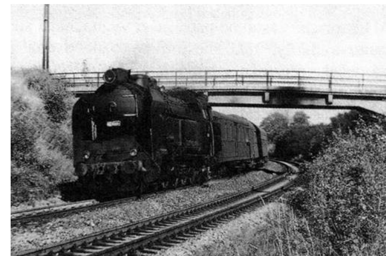
Fig. 6 Historical photo Black Bridge, source: nasepraha.cz
