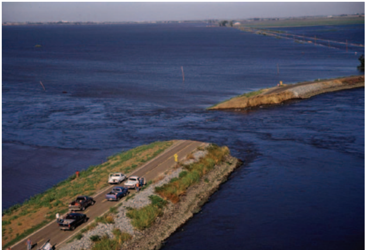
Levee Failure
