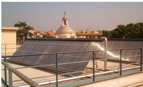
Figure 3.13: Evacuated tube solar thermal collectors. Image: [60].
