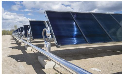
Figure 3.12: Flat plate solar thermal collectors. Image: [59].
