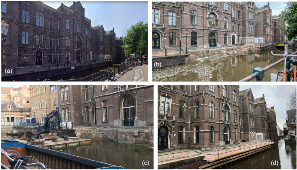
Figure 3.1.: Collapse and reconstruction efforts at the Grimburgwal canal in Amsterdam (area highlighted on Fig. 3.2 by a black rectangle). (a) Before collapse. (b) Aftermath of collapse [GA1, 2020]. (c), (d) Reconstruction efforts.
