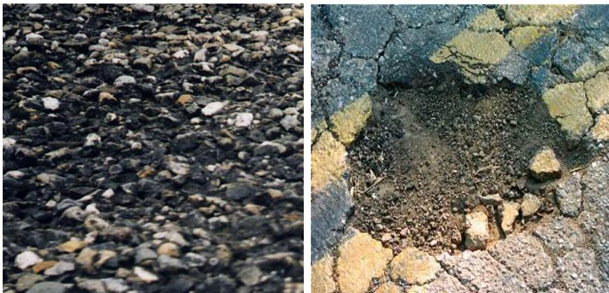
Fig. 1.1.1: Moisture induced damage in asphalt (a) raveling (b) potholing
