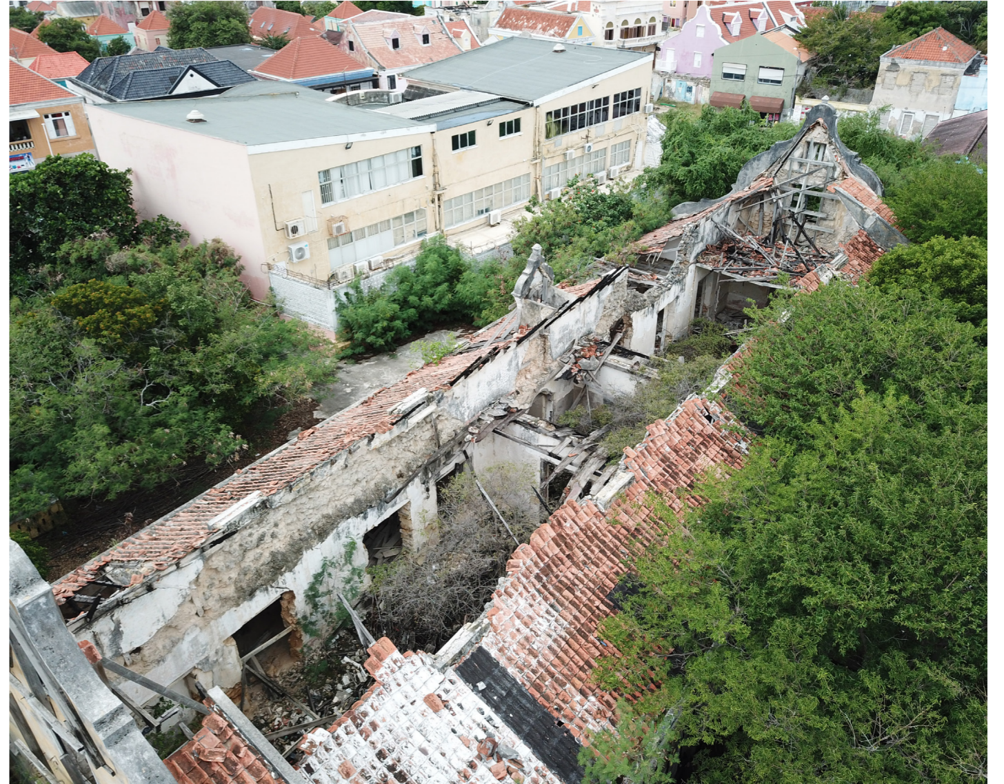
Drone shot current state of manor house envelop
