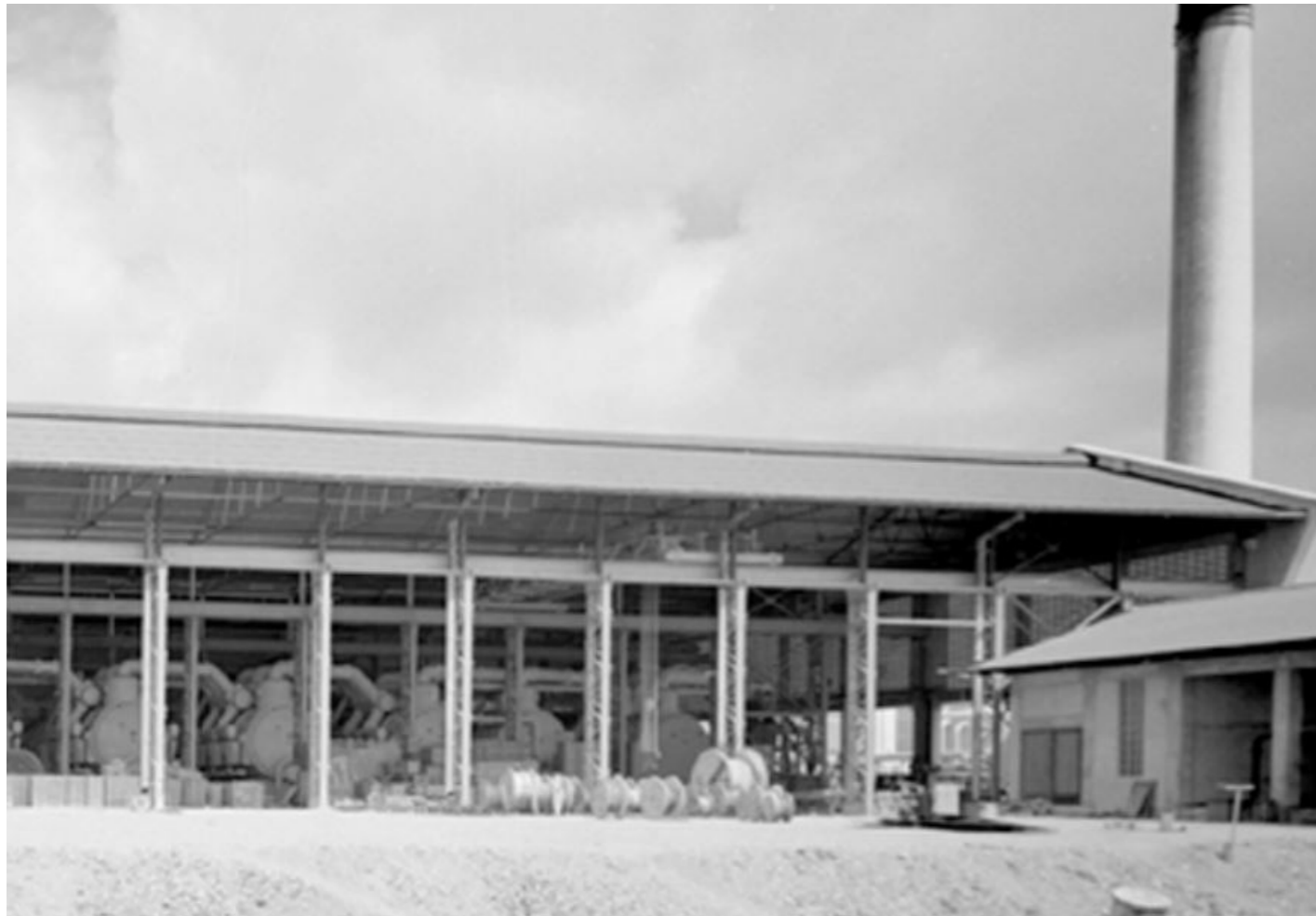
Reverse-osmosis plant Aqualectra
