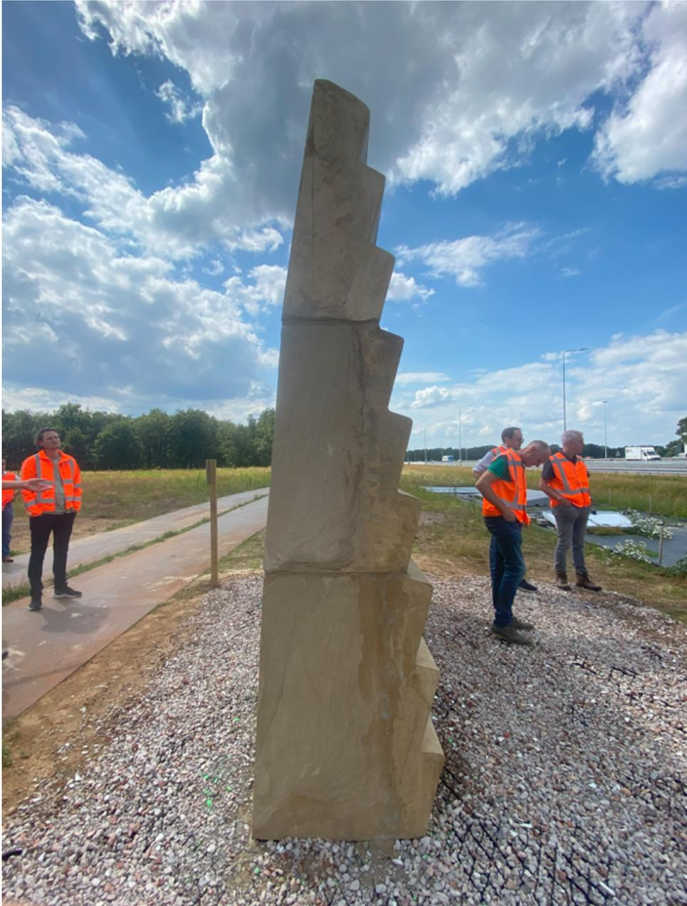
Figure 3.21: Sustainable noise barrier built at the InnovA58 site
