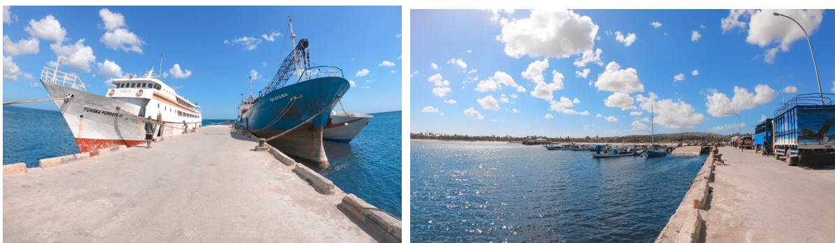
Figure 36. View of the Port of Seba in East Nusa Tenggara, Indonesia (Courtesy of Ministry of Transportation, 2019)
