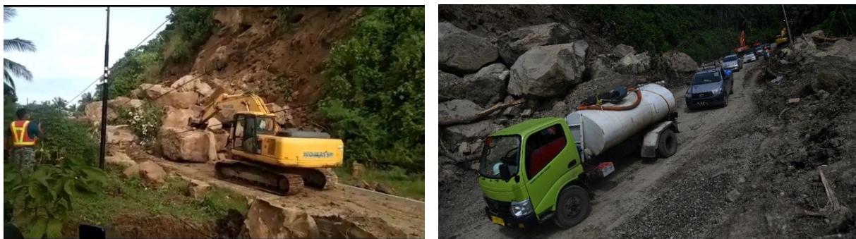
Figure 68. A road section on route 2 was completely blocked by landslides, making it impassable for vehicles (a); A road section on route 1 that was affected by landslides but remains passable for vehicles (b) (Courtesy of detik.com)
