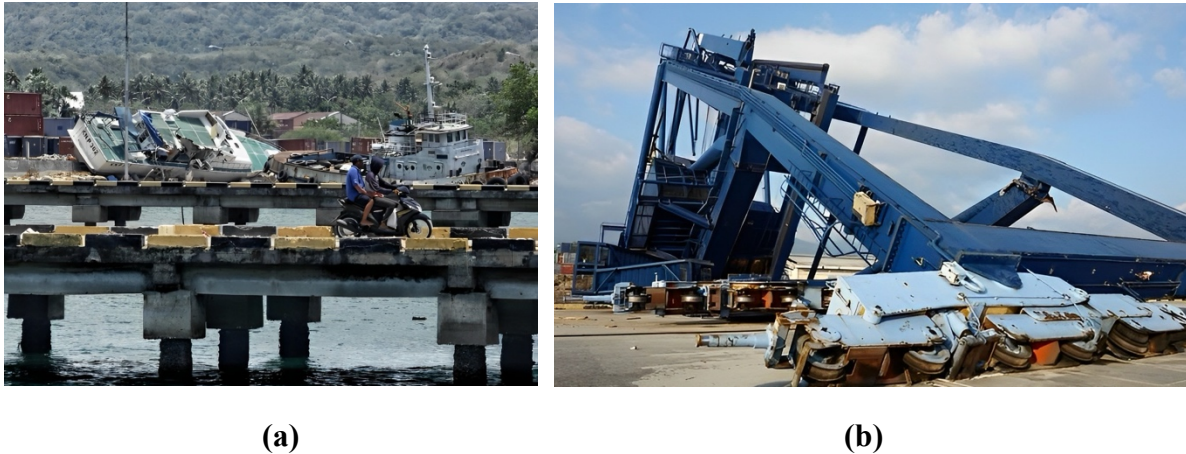
Figure 29. Ships were stranded at the dock, preventing other ships from accessing it (a), and the quay crane collapsed at the Port of Pantoloan (b) (Courtesy of PT. Pelindo)
