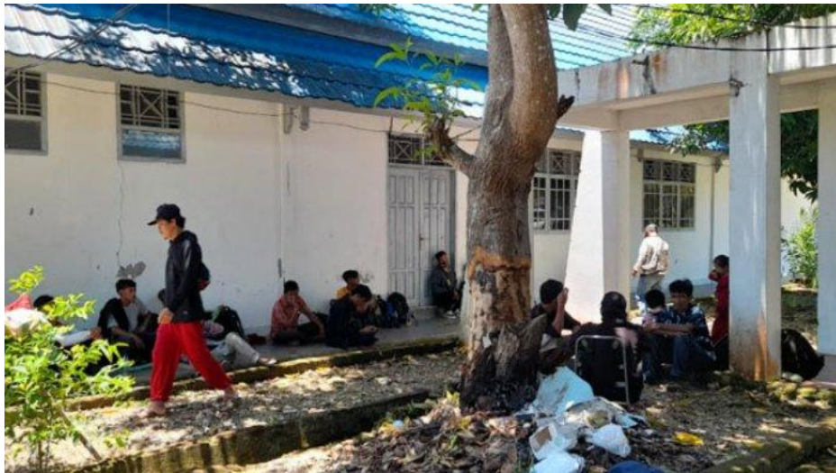
Figure 70. Mamuju Simboro Port passengers await on the passenger terminal platform amidst ongoing landside facility rehabilitation (Courtesy of Tribun-Sulbar news agency)
