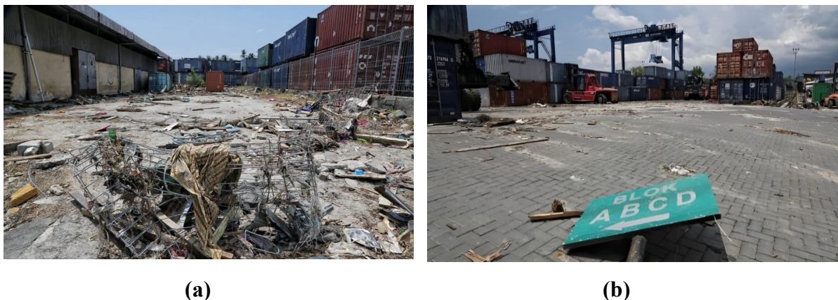
Figure 30. Condition of the partial stacking yard area affected by tsunami (a), and condition of the other partial stacking yard area that can still be used (b) (Courtesy of PT. Pelindo IV)
