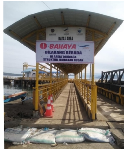
Figure 64. 10 cm displacement of the trestle and berth connection (a); Warning sign for passengers to avoid the berth area due to damaged trestle of bridge structure (b)
