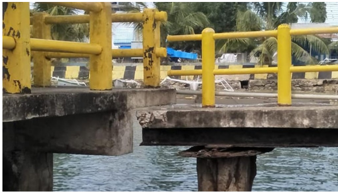
Figure 64. 10 cm displacement of the trestle and berth connection (a); Warning sign for passengers to avoid the berth area due to damaged trestle of bridge structure (b)
