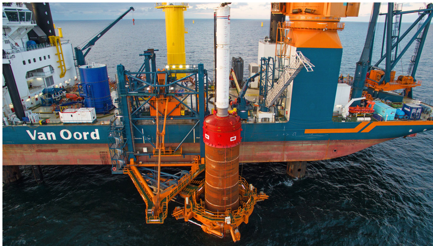
Figure 3.18: Pile driving of a monopile [18]
