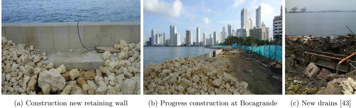
Figure C.1: Construction of new pedestrian promenade at Bocagrande and Castillogrande
