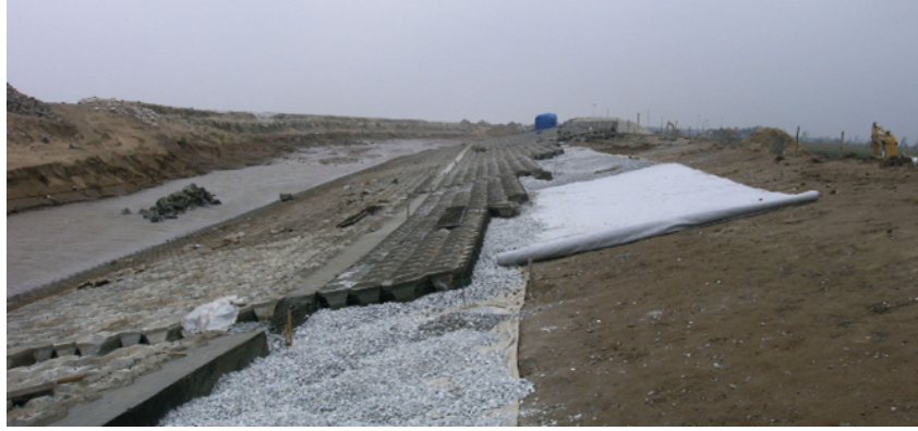
Figure 8.16: Different construction stages of a revetment in one picture
