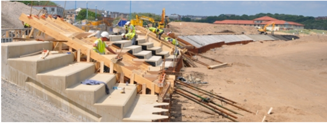
Figure 8.15: Construction stages of the promenade [28]
