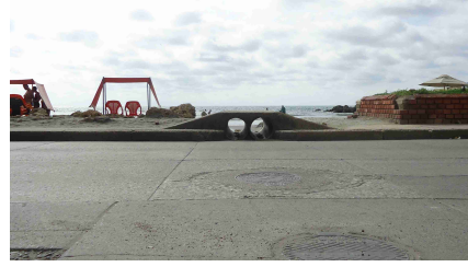
(b) Insufficient drainage: Open drainage to the sea
