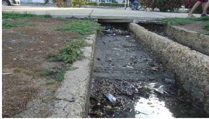
(c) Insufficient drainage: garbage in drains
