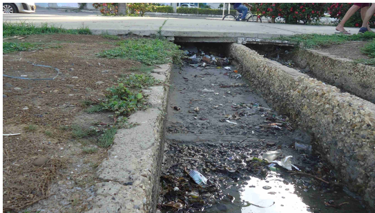
(e) Clogged outlet drain
