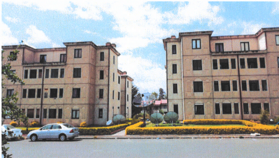
Figure 19: View of residential apartments at the CMC compound.
