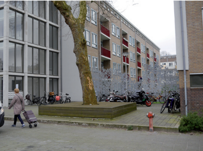
Fig.5.43 Renovation of the Dudokhaken: addition of storeys, staircases and re-framing the space by fencing off the open courtyards (Photo: author)
