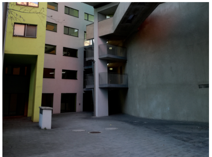
Fig.5.27 Dark corners in the Kabelwerk Meindling (Photo: author)
