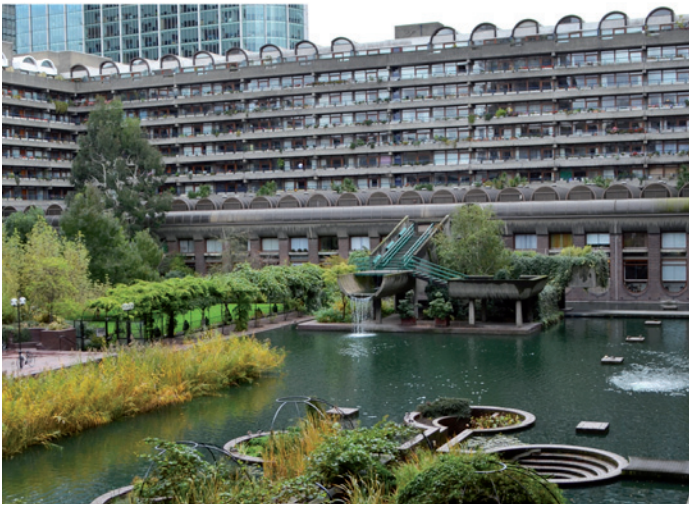
Fig.4.6 The Barbican, London's most iconic brutalist ensemble (Photo: Photographer unknown, retrieved from ArchCentre, 2016)
