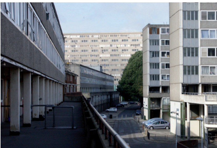
Fig.1.6 Deck access pathways at the Aylesbury Estate (Photo: retrieved from terrainsurveys.co.uk , 2014)
