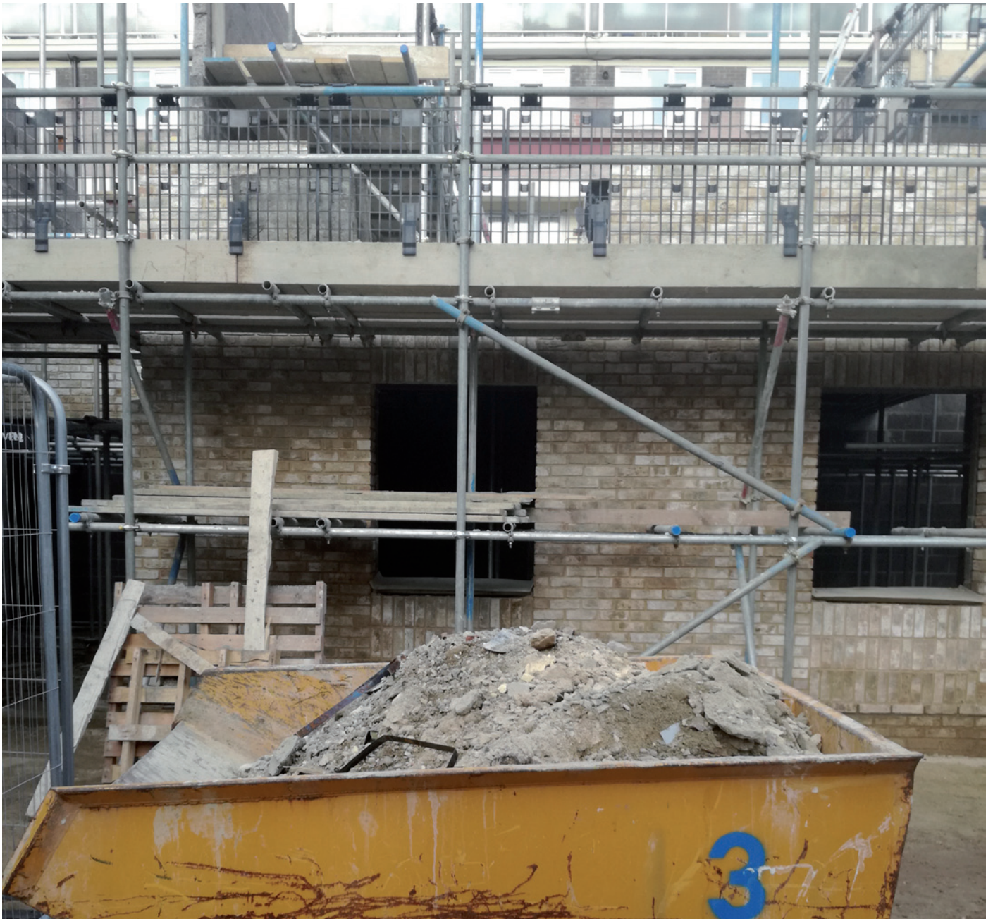
Fig.4.68 Construction of the infill sites is under way (Photo: author)
