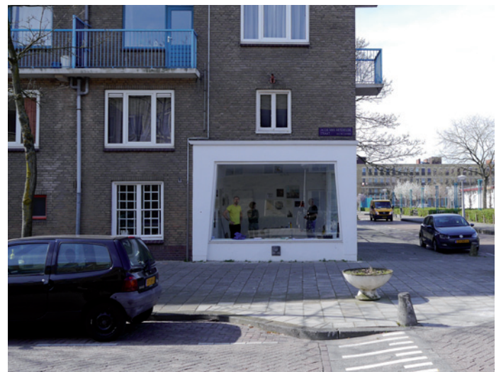
Fig.5.46 Renovated cornershops enliven the street, also Kolenkitbuurt (Photo: author)
