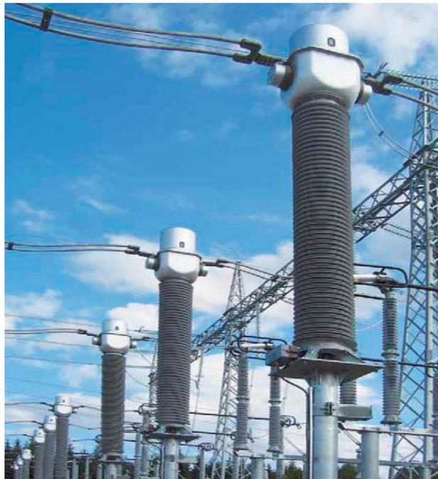
**Figure 3-1.** Typical current transformer used in HV applications [Source: [www.directindustry.com](http://www.directindustry.com)]
