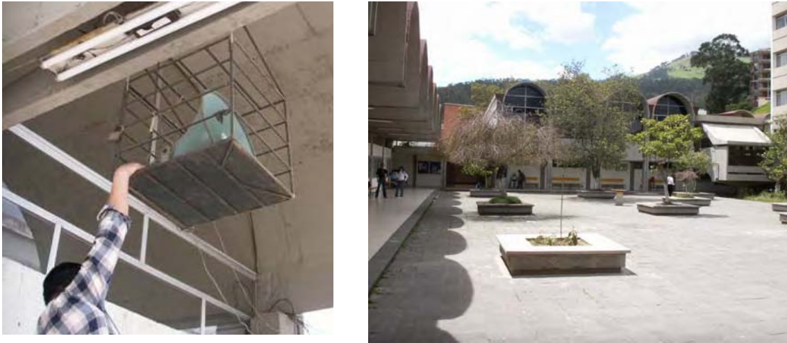
Figure 11.1. Central square of the Faculty and location of the sensor.
