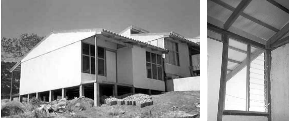
Figure 12.1. External and internal view of the house selected for temperature measurements, seen from the South.
