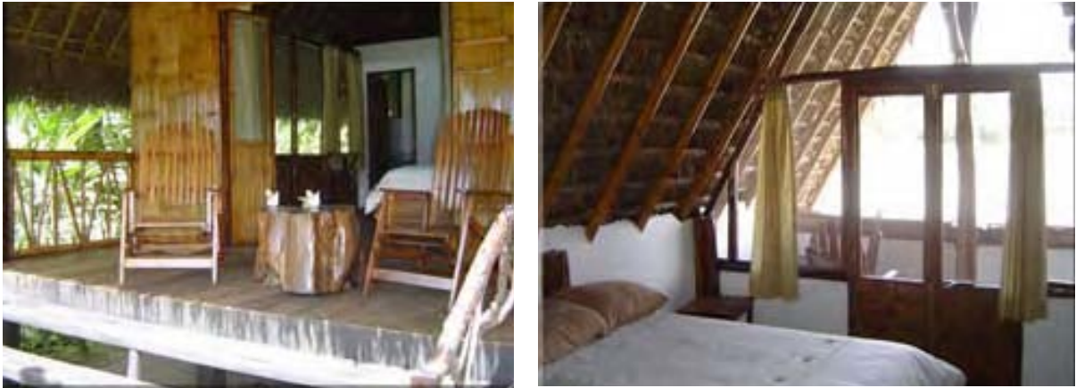
Figure 12.8. Cotacocha, Napo, Ecuador, traditional construction with cross ventilation.
