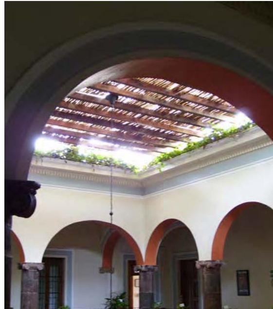
Figure 11.31. Moderation of the high light levels.
