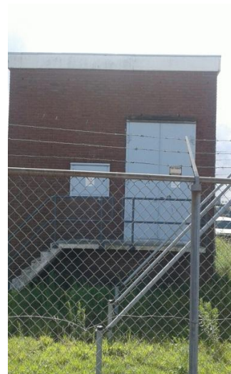
Figure 3-2 Elevated electrical station (personal photo)
