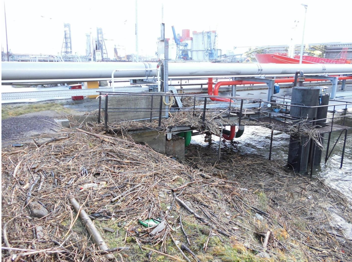
Figure 2 Flood at terminal Neuhof
