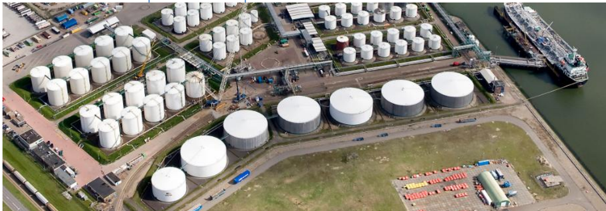
Figure 4-2 Part of the terminal of Chemiehaven (Vopak archive)
