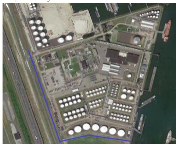
Figure 4-39 Terminal Scale; Flood wall or Ditch at the Terminal Chemiehaven
