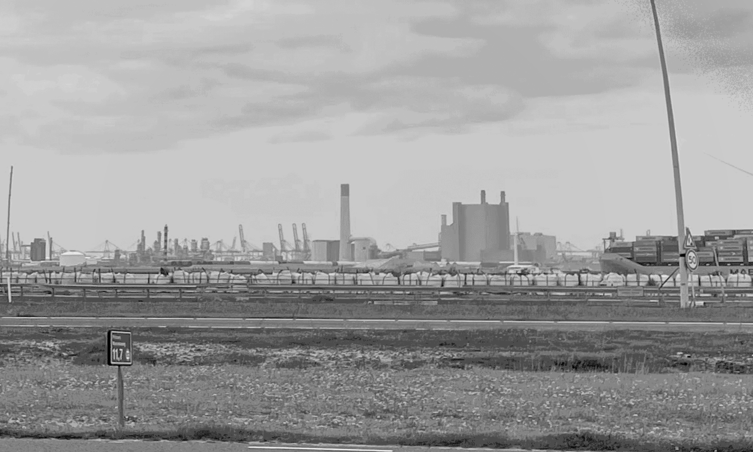
Facilities in the Maasvlakte, the Port of Rotterdam Source: Photo by author, 2021
