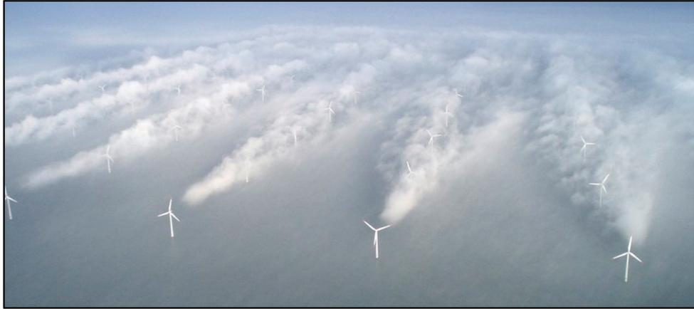
Figure 1.2.: Wake visualization in the Horns Rev offshore wind farm located in Denmark. The wakes are visible as vapour trails, clearly showing that a wind turbine can be the wake of multiple turbines resulting in a cumulative reduction in wind speed. Photographer: Christian Steiness (February 12<sup>th</sup>, 2008) [12].
