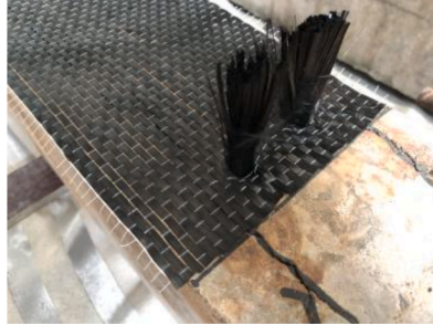
(b) CFRP anchors inserted into concrete
