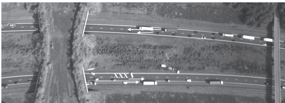
Figure 9.2: The incident location near Apeldoorn (A1). The three white X's indicate where a lane blockage was present.
