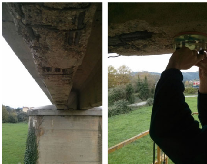
Fig. 2 Selected areas during the repair phase
