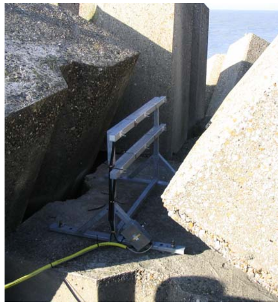
Figure 36: Velocity meter in front of pipeline.
