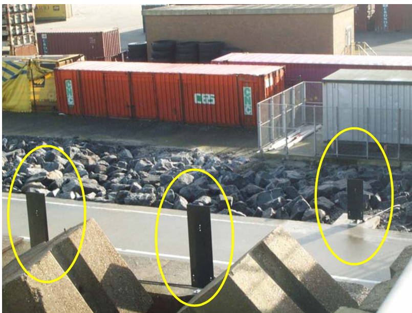
Figure 31: Global view showing three installed instrumented dummies on site.
