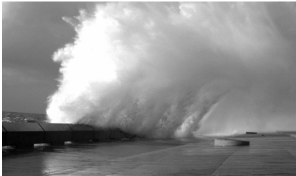
Fig. 9: Violent wave overtopping at Samphire Hoe (Picture courtesy of Eurotunnel and the White Cliffs Countryside Project).
