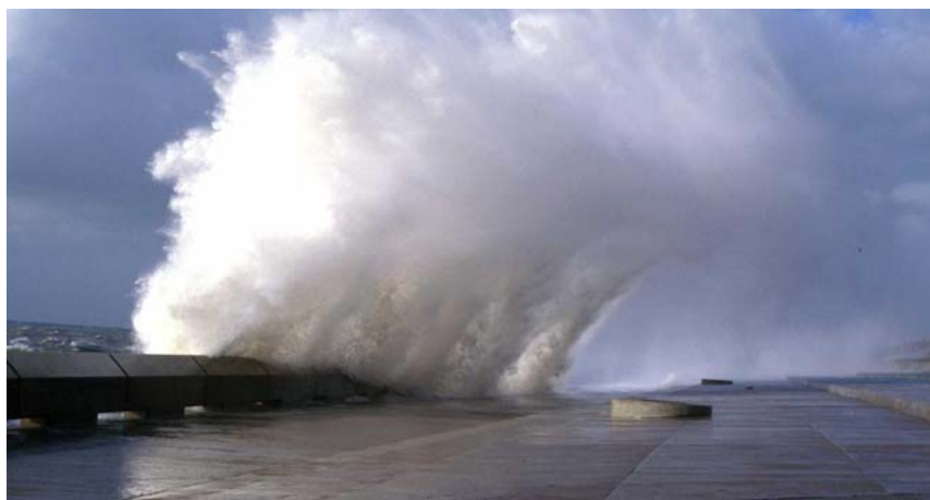
Figure 53: Violent wave overtopping at Samphire Hoe (Photograph courtesy of Eurotunnel and the White Cliffs Countryside Project)
