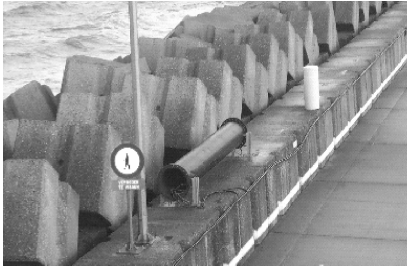
Figure 32: Global view showing the instrumented pipeline on site.
