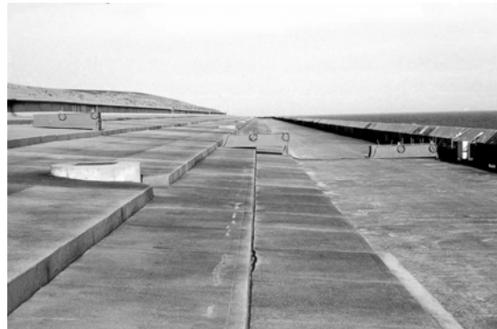
Fig. 10: Overtopping tanks at Samphire Hoe.
