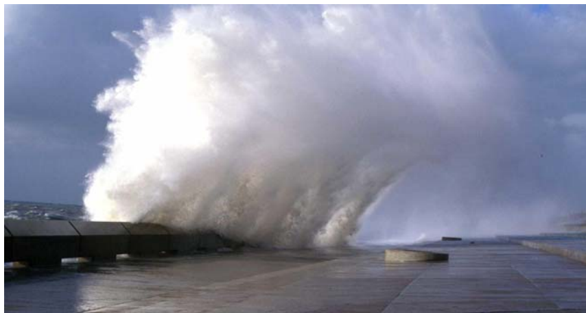
Figure 53: Violent wave overtopping at Samphire Hoe (Photograph courtesy of Eurotunnel and the White Cliffs Countryside Project)
