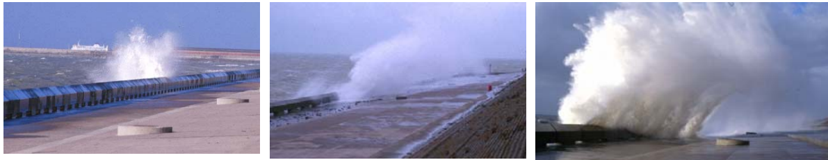
Figure 100: Categorisation of overtopping hazards at Samphire Hoe, low, moderate and high
