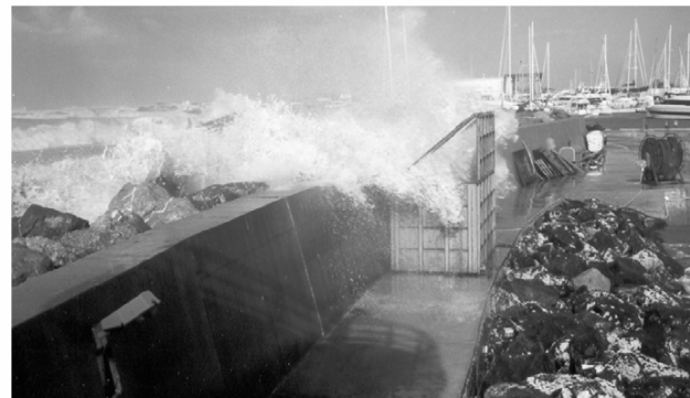
Fig. 7: Wave overtopping in the tank at Ostia.
