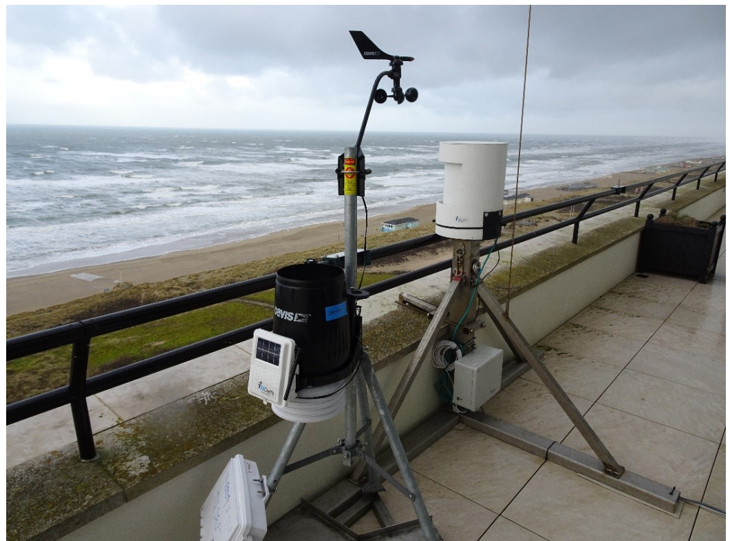
Figure 1. TLS and the weather station installed on the upper balcony of the Huis ter Duin Hotel, Noordwijk, the Netherlands.
