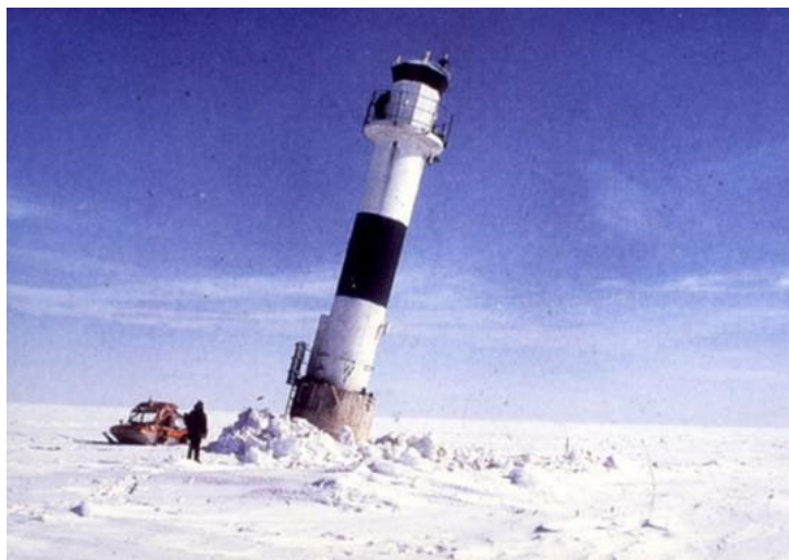
Figure 1. The Swedish lighthouse Björnklacken after being displaced by sea ice in 1985 (photo by Lennart Fransson).
