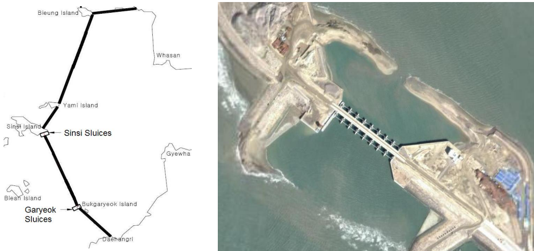
Figure 1.3: left: location of sluices; right: Garyeok sluices during construction
