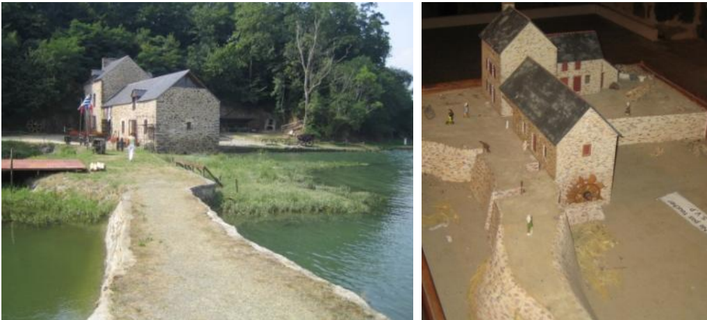
Figure 2.2: 19 th century Moulin du Prat (left) and scale model of Moulin du Prat (right)
