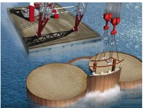
Figure 5.12: Installing spandrel walls
