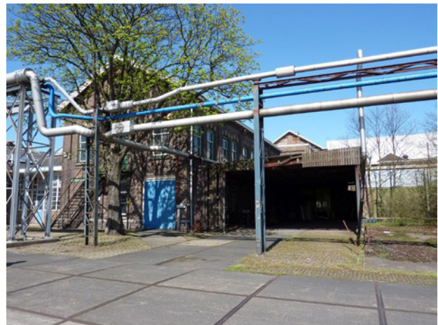
Figure 3: Demolished building 513 , with wooden structure (Steenhuis & Meurs, 2010).
