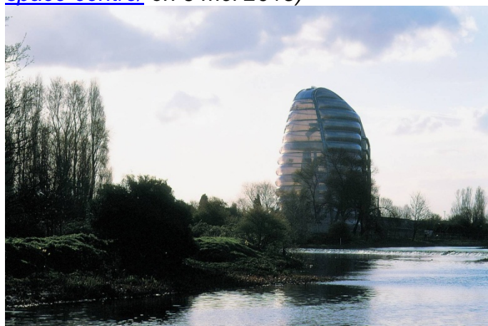
Figure 11: view to the buidling (Grimshaw architects)
