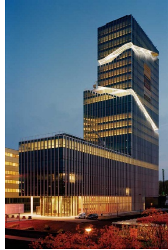
Figure 14: Vinoly tower source: http://www.e-architect.co.uk/holland/mahler4-office-tower
