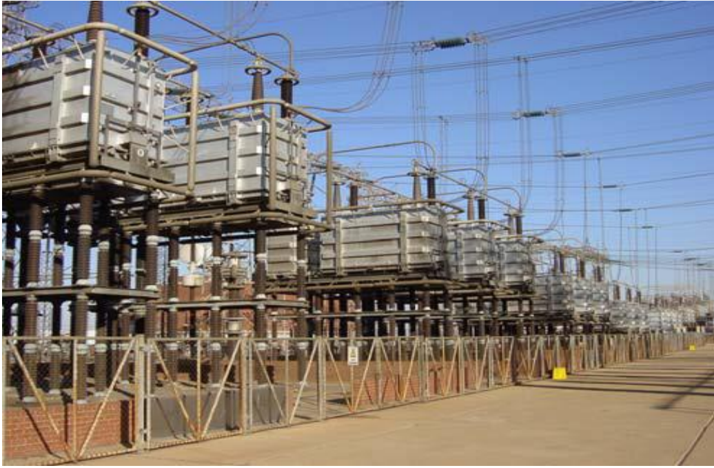
Figure. 3.1 Outdoor thyristor valves immersed in oil at Apollo HVDC station [40]
