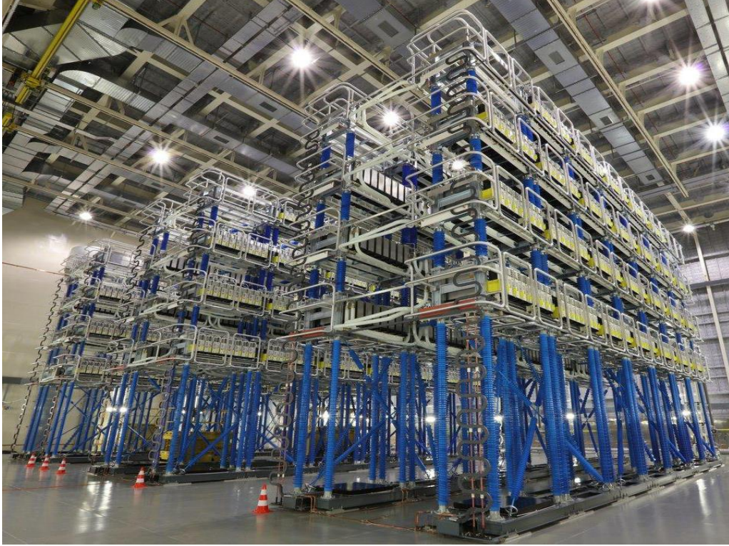
Figure 2.15: Internal view of the converter valve hall (Alstom Grid) with type II connection [27]
