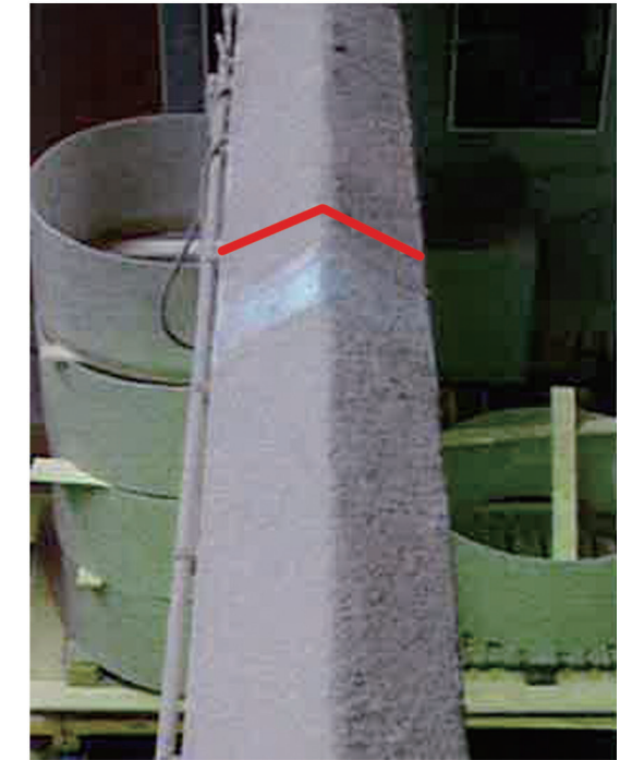
fig3. The sloped top surface of the beams without walkways on them.(marked in red)
