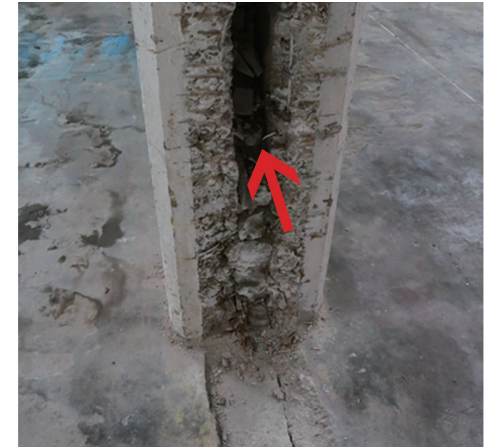
The cavity between compartment walls
