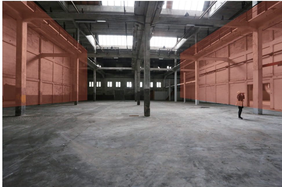
The compartment walls viewed from the interior
