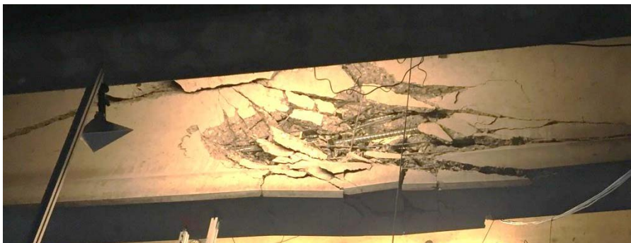
Figure 8 Shear failure beam test 1
