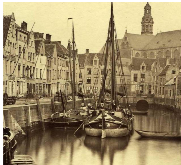
FIGURE 2.1.9: (Top) A historic sketch of the Suikerrui and the Boterrui, the canal used as a trade artery, specifically for trade of sugar and butter products imported by ship (FelixArchief, n.d.). (Bottom) A photograph of the Koolvliet, known today as the Koolkaai, showing coal ships moored in the inner city (HLN, 2016).
