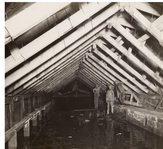
FIGURE 2.1.10: (Top) A diagram of how the canals were enclosed by a vaulted tunnel after they became overused as open sewers (The Ruien Antwerp, n.d.). (Bottom) A photograph of the construction of a vaulted ceiling on top of the unknown section of canal (FelixArchief, n.d.).
