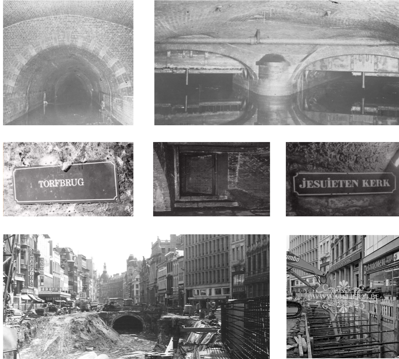
^ FIGURE 3.2.2.15: (Top left) Differently vaulted ceilings, arched in foreground and pointed in background. (Top right) A sluice construction at a tunnel junction. (Middle) Historic street signs (left and right) act as silent guides for the secret passages from above (center). (Bottom left) An historic bridge exposed during the 1975 construction of the metro station at the Meir. (Bottom right) Construction of a rectangular tunnel made of concrete to bypass the new metro station.
