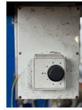
Figure 3.7: The three way valve temperature button, not calibrated.
