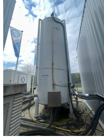
(b) The warm 20 m 3 vessel, outside, without insulation.
