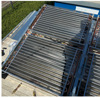
(b) Topview of the thermal collectors installed, the Alius EVO
