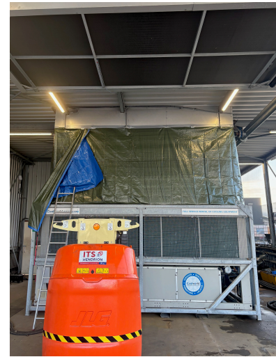
(c) Sail is now fully enclosing the cooling machine.
