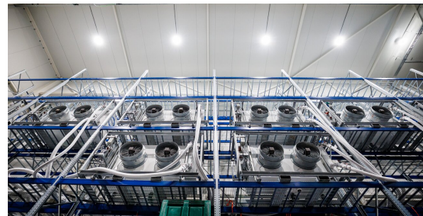
(b) Air handlers inside of warehouse
