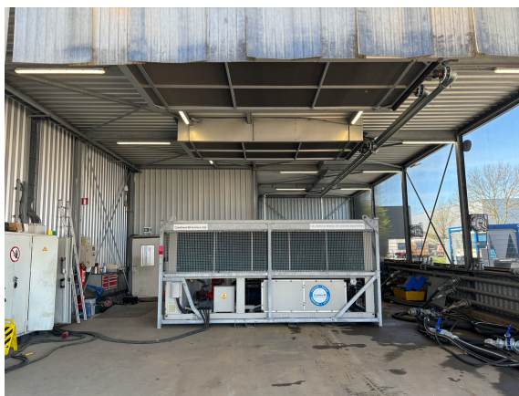
(a) Cooling machine positioned under heat exchangers
