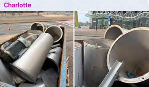
Old ventilation pipes
