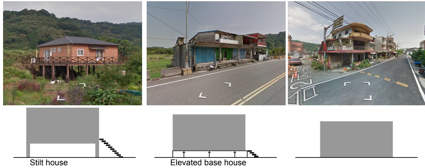
Figure 3.31 The local dwelling has developed few housing types to adapt the living condition with flood. 1) Stilt house in high flood risk area, 2) elevated base house in mid flood risk area, and 3) normal housing type in low flood risk area.
