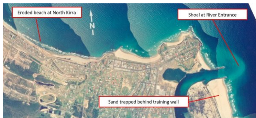
Figure 5.2: The Tweed River Entrance before the construction of the sediment bypass system. The sedimentation behind the training wall and at the river entrance and the erosion at North Kirra are indicated. (Tweed Sand Bypassing, 2020)
