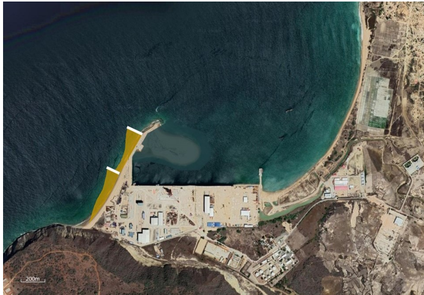
Figure 4.19: Strategy 3 - Blocking structure: groynes
