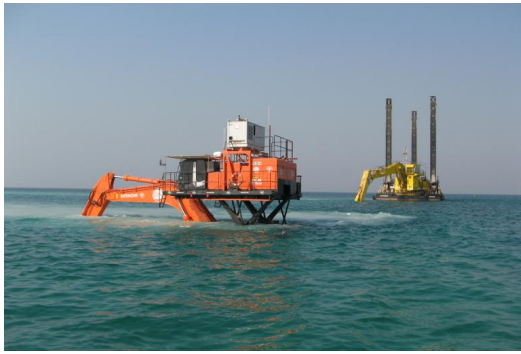
Figure 2.1: Operating BHD and EEX in the nearshore zone (jandenu.com, 2021)
