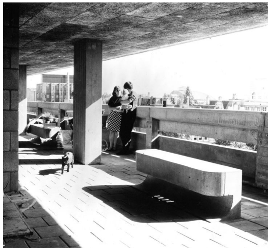
Concrete lighting blocks, Weesperstraat student housing
