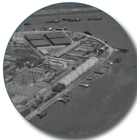
Demolishing of long Marine shed
