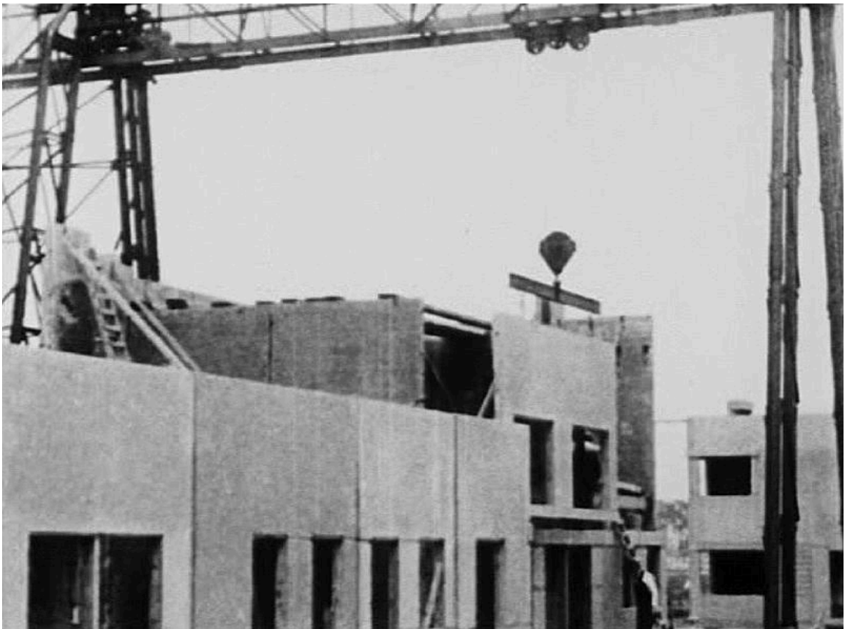
Image 10 Betondorp construction site and assembling of pre fab panels https://www.betondorp.org/Slideshow/slides/A20.html
