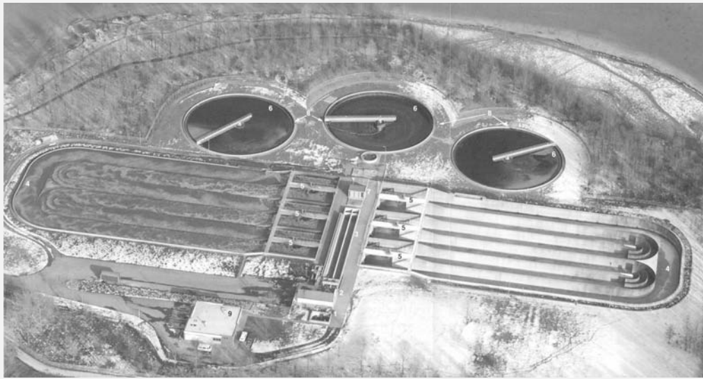
Figure 2-C.2 Treatment scheme of wwtp Kaffeberg; see text for the explanation of the numbers
