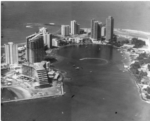
Figure C.21 Around 1981 - Just after the building of the Hilton. No tennis fields and pool yet
