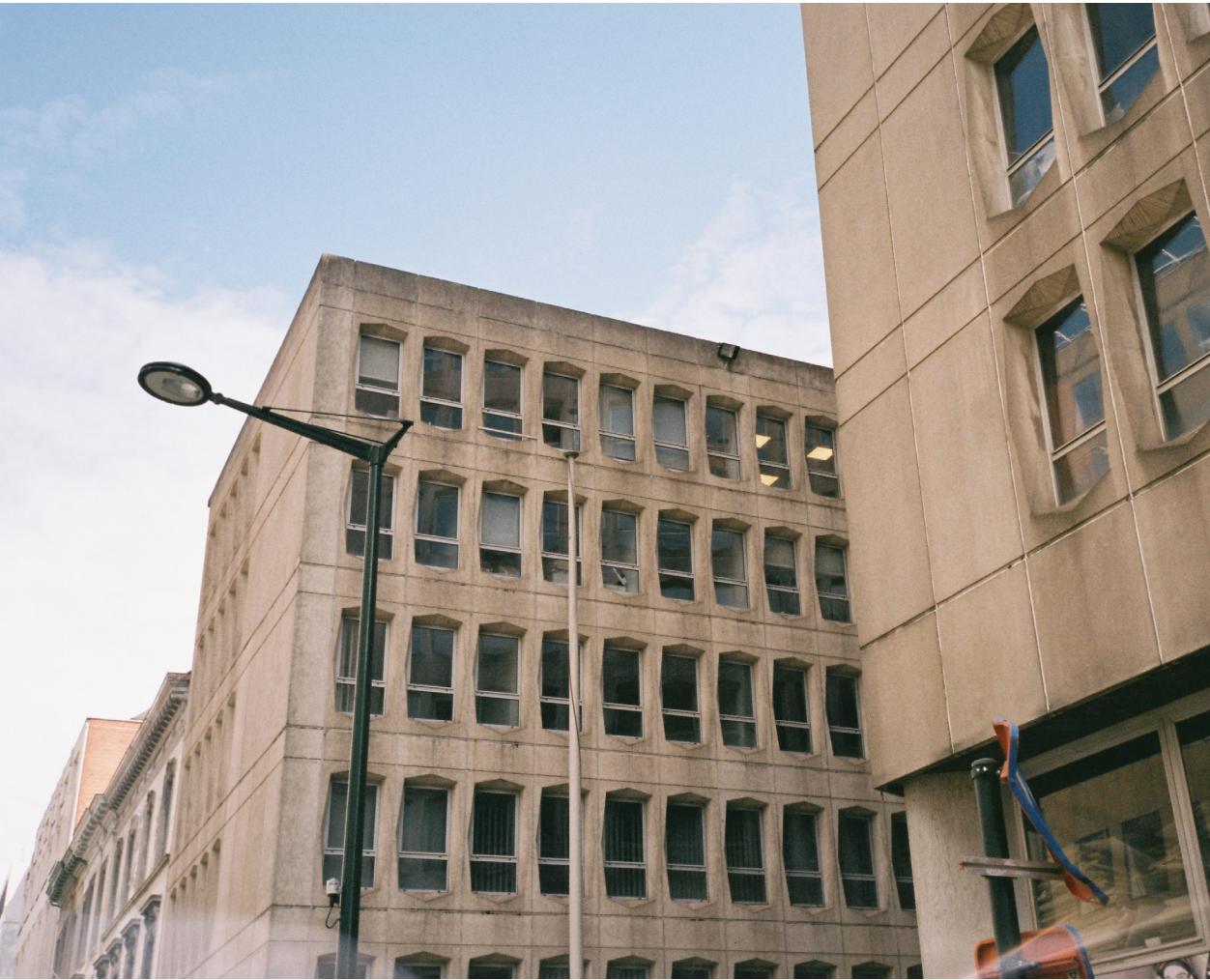
Fig. 1.1: Rue de la Loi, Brussels Photograph by Max Schuska
