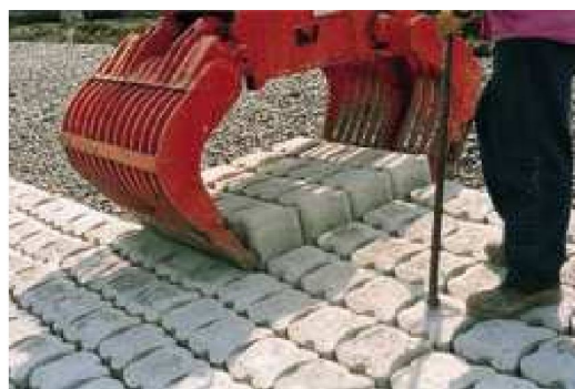
Figure 1.2: Placing of Hydroblocks, from (Dorst et al., 2012).
