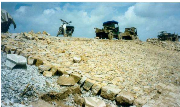
Figure 1.1: Pattern placed revetment with shaped natural rock, from (Dorst et al., 2012).
