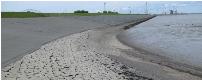
Figure 3.1: A dike along the Wadden Sea with both a placed block revetment and asphalt on the top layer.
