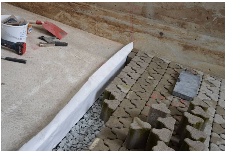
Figure E.2: C-star revetment
