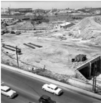
Tunel de La Habava in construction
