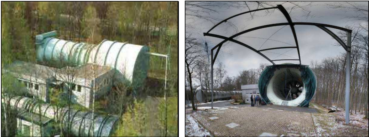
Figure 5.2: Aerial view [Source: Böenwindkanal] and front view of the Böenwindkanal.
