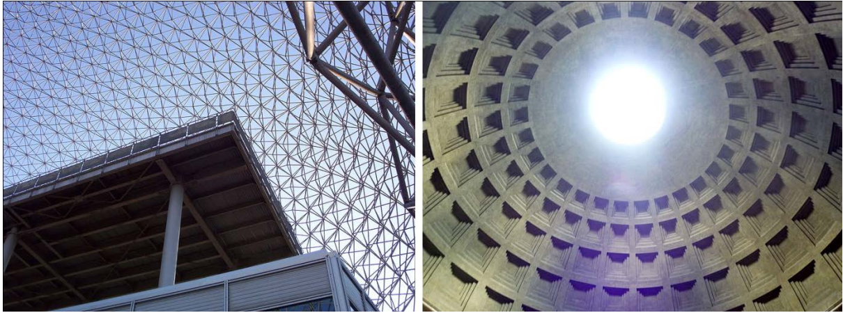
Figure 1.5: Domes as a comparison of elementized, Montreal Biosphère (left) and monolithic construction, The Roman Pantheon (right) [Colocho, Fczarnowski].
