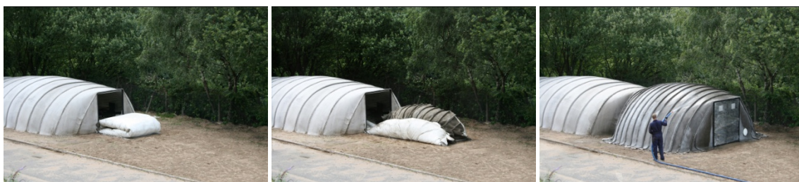
Figure 3.3: Erection procedure of the inflatable Concrete Canvas Shelter. [Concrete Canvas]
