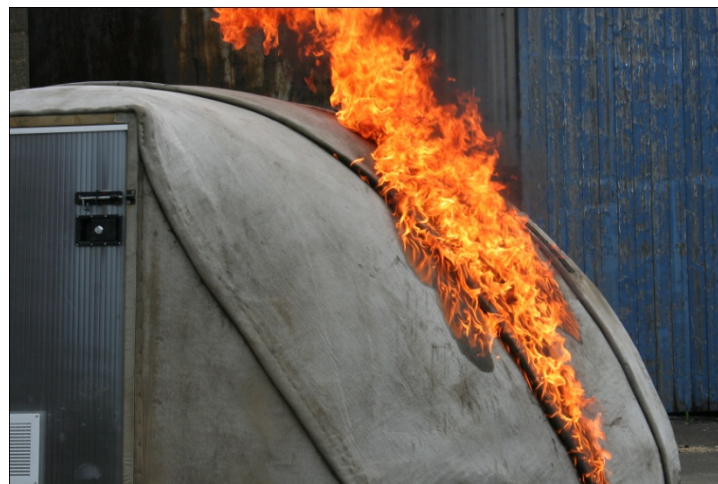
Figure 7.2: Concrete Canvas Shelter with localized external fire. [Concrete Canvas]
