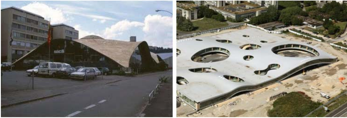
Figure 1.7: Examples of high, structurally efficient, curvature, Sicli Company building (left) and a thick low curvature, load bearing surface, Rolex Learning Center (right) [Unknown1, Epfl Alain Herzog].
