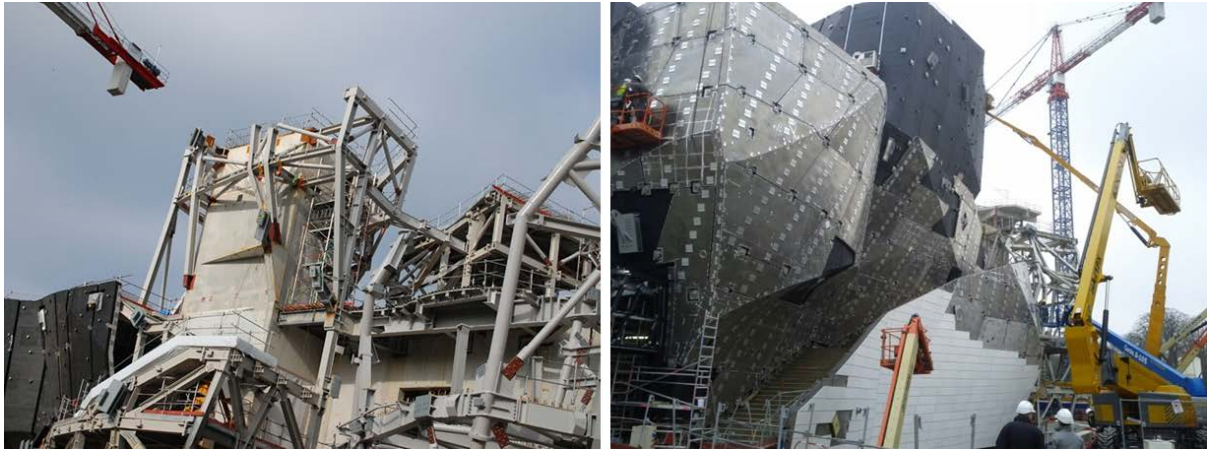
Figure 1.3: Louis Vuitton Foundation, before and after cladding [Piéton, Kapoutrocknroll].
