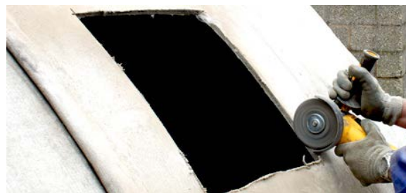
Figure 3.4: Hole cut into Concrete Canvas Shelter. [Concrete Canvas]
