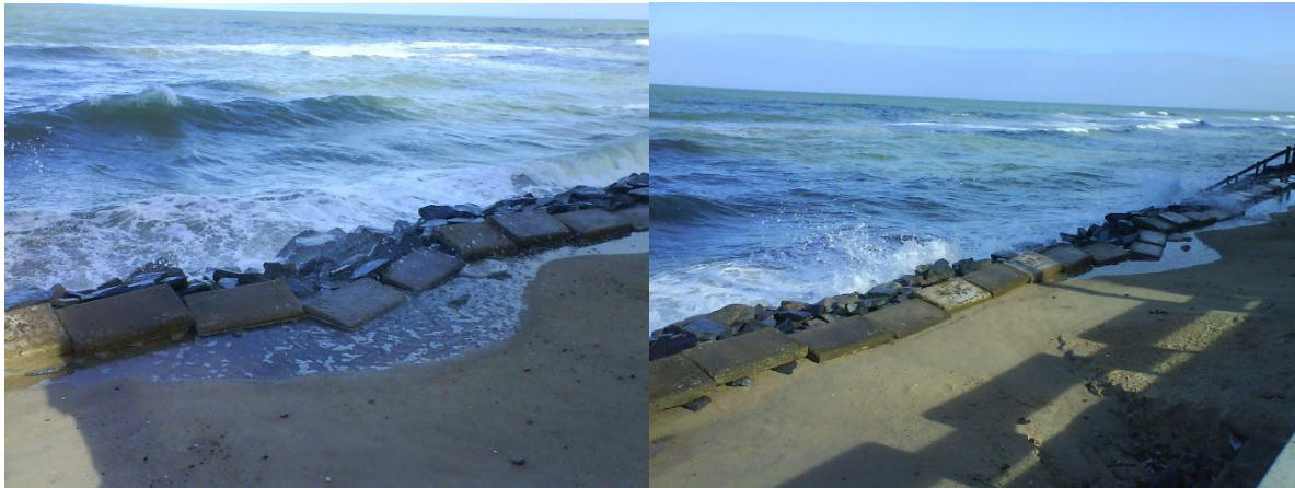
Figure 45: Overtopping during high tide at revetment E
