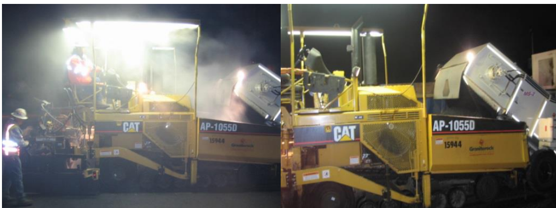
Fig. 4. Fumes from HMA (left) and high transparency from WMA (right) (Jones, 2013)
