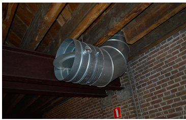
13. floor and beams cut off for placement of a ventilation shaft
