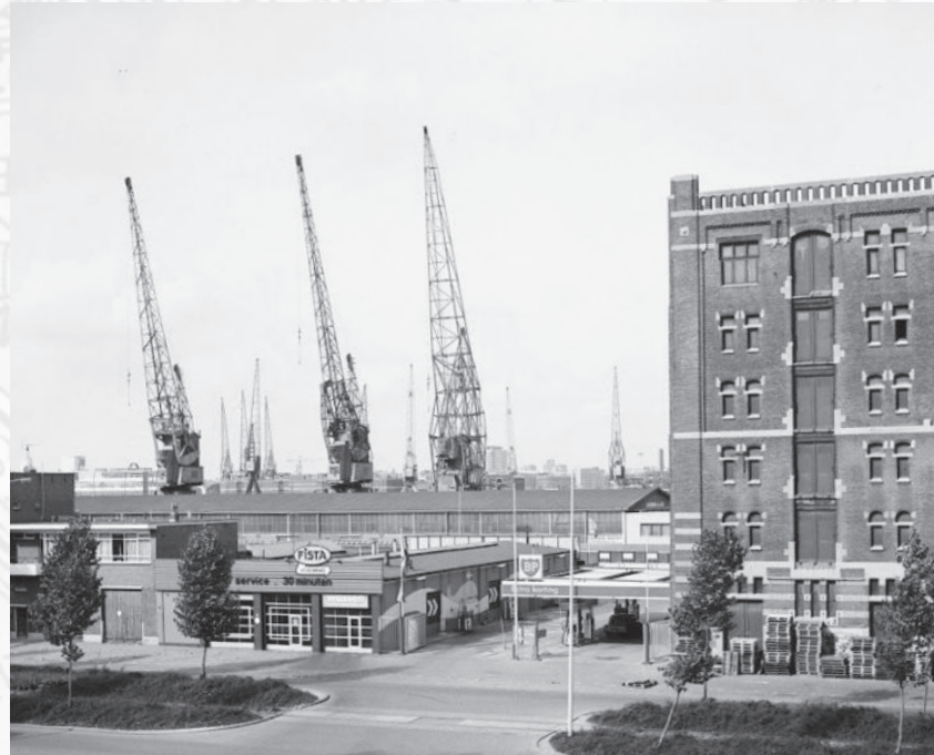
south facade, during this time there was a tank station attached to the west side of the building. wench houses are gone.
