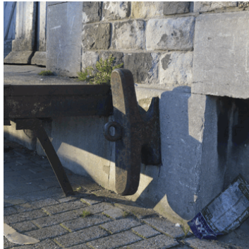
1. T-shaped metal piece to which ropes can be attached. possibly used for the ropes from the wenchies.
