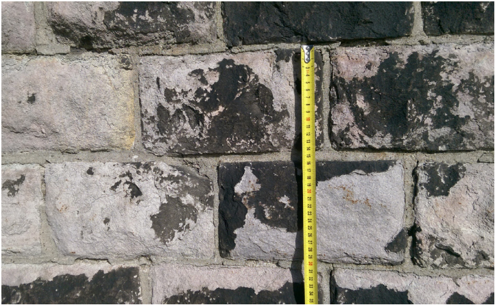
photo 2: height of a stone is aprox. 140mm pointing is aprox. 20mm thick
