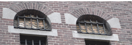
4. Filling of the top windows on the 1st floor with brickwork
