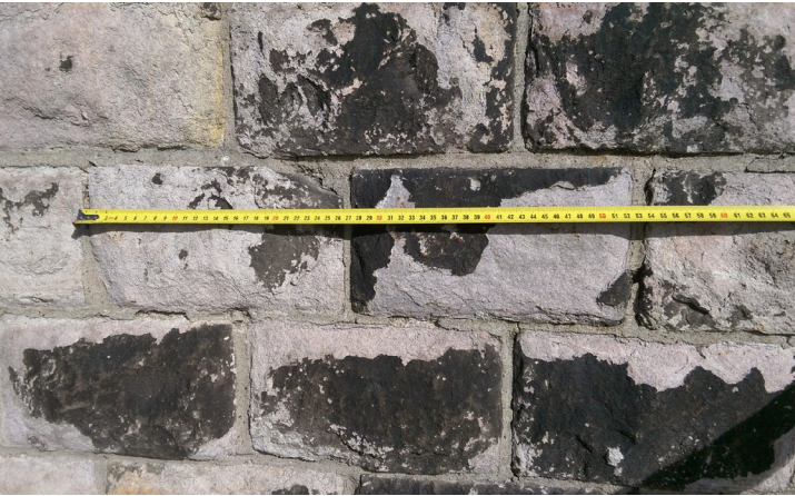
photo 1: width of a full stone is aprox. 250mm / joint is aprox. 10 mm thick
