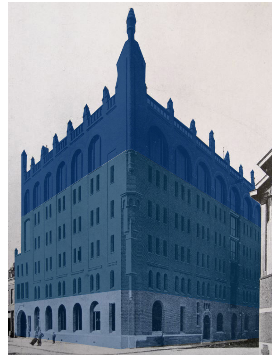
Image 3: Vd Lugt: division of the facade into the plinth, the middle and the attic zone
