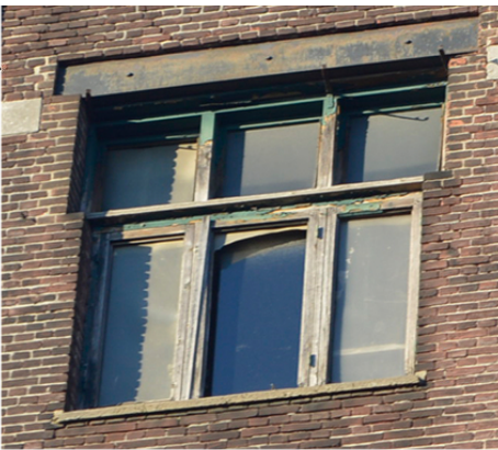
10. Replaced window on the 5th floor
