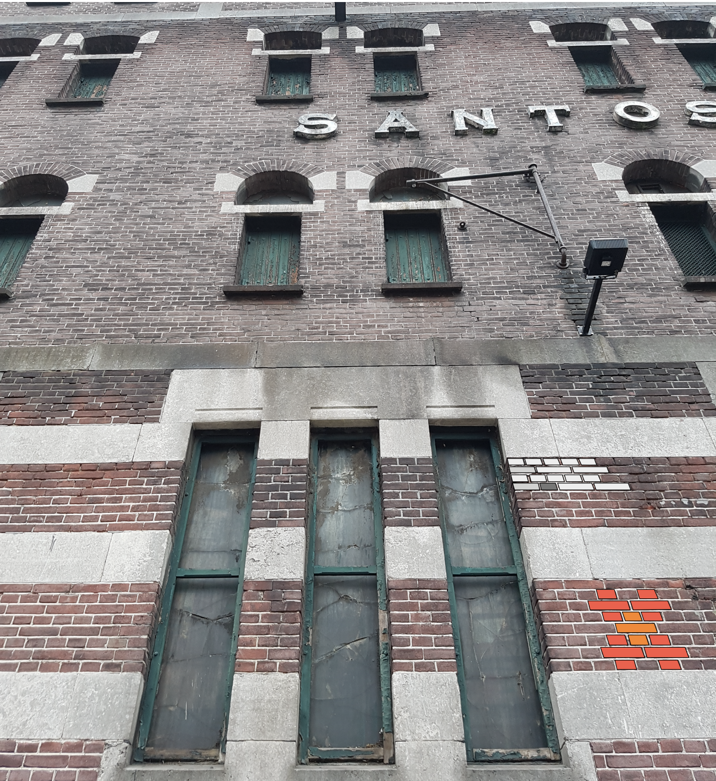
photo 1: brick masonry bond in Santos
