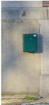
6. Filling of the basement entrances and windows with brickwork and finished with a concrete plaster
