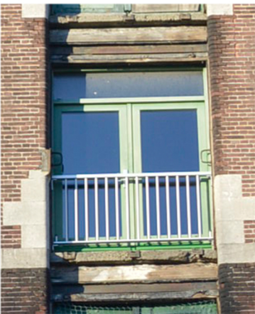
3. Filling of the 3rd floor door openings with glass doors and a metal railing
