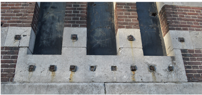
5. Removal of the metal safety bars on the ground floor windows
