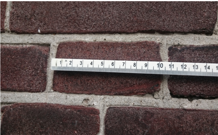
photo 1: width of a half stone is aprox. 100mm pointing is aprox. 10mm thick
