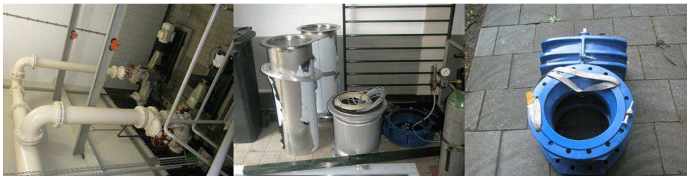
Figure A.3: Flow sensor (electromagnetic flow sensor OPTIFLUX 2000) at the pumping station in the 'Tuindorp' sewer catchment (Professor Leonard Fuchslaan). Installation of the flow sensor followed the standard EN 287/EN ISO 15614 (Welding) and has been calibrated against a fixed-volume tank.
