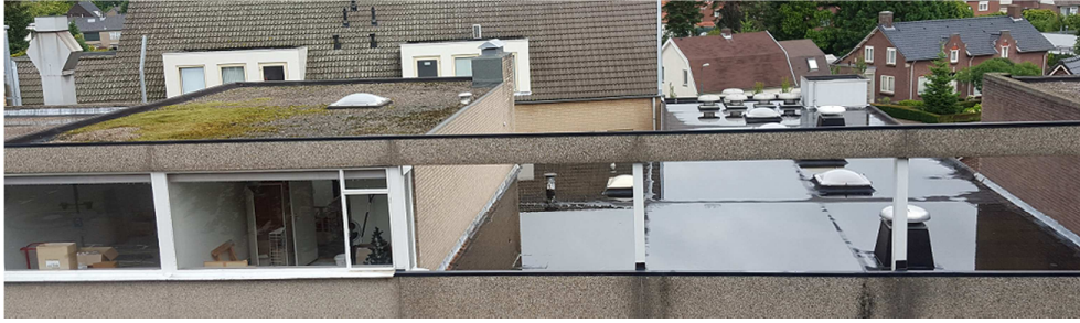
Figure 3.7: Local hydrological circumstances on roofs affecting total amount of runoff water (vegetation and storage).
