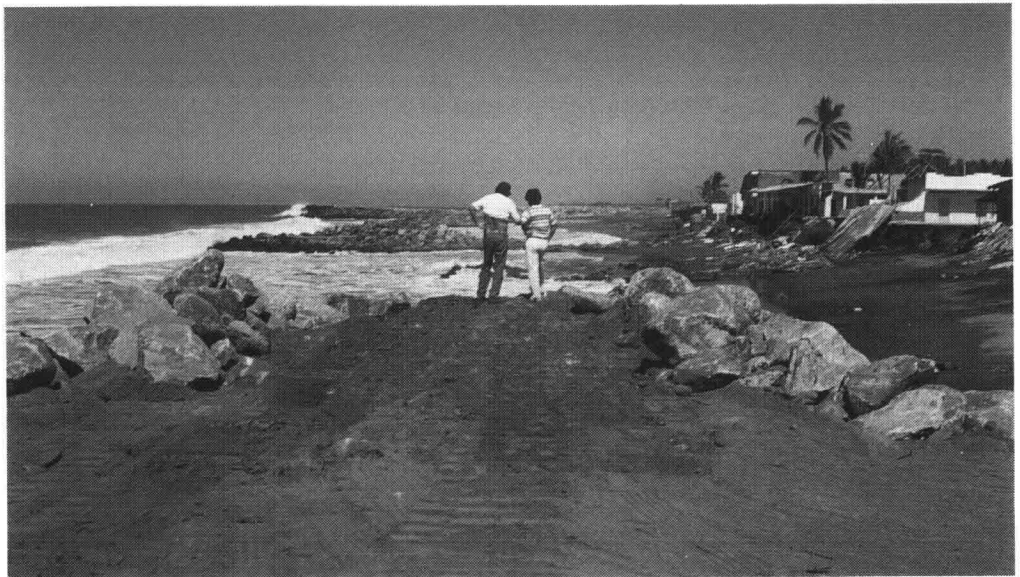
Fig. 4-3 Sea-wall in process of construction within groin of No.13 to 16
