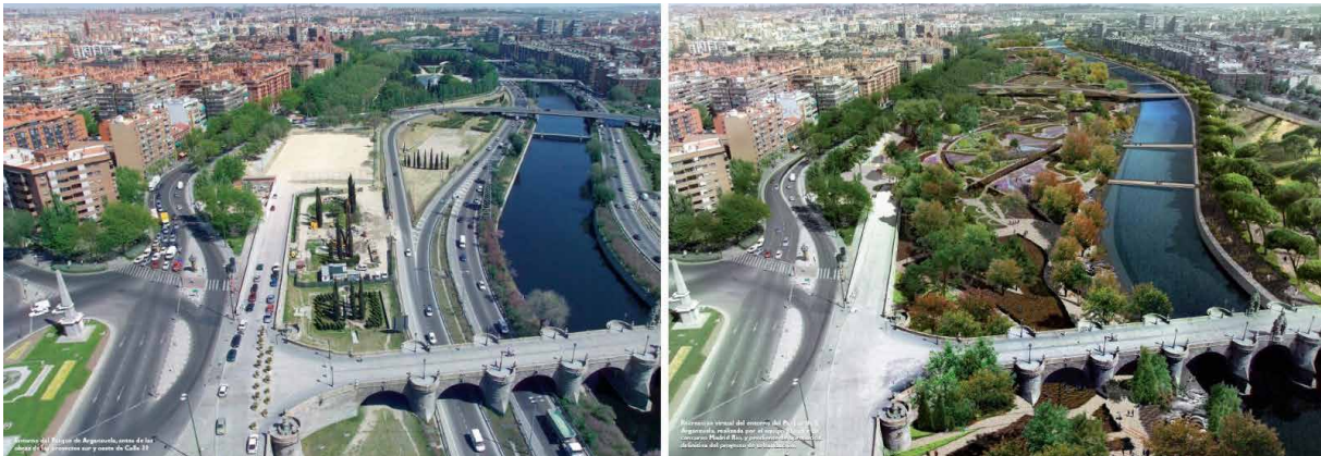
FIGURE 7.15 River Manzanares before and after the Madrid Río project. Source: eoi.es. Retrieved from: http://www.eoi.es/blogs/imsd/project-management-rio-madrid-project/ (Accessed: 1 August 2018).
